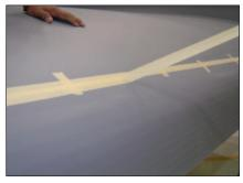
Installation of tape to be used as a hinge for the  $3M^{\mathbb{N}}$  Polyurethane Protective Tape.
